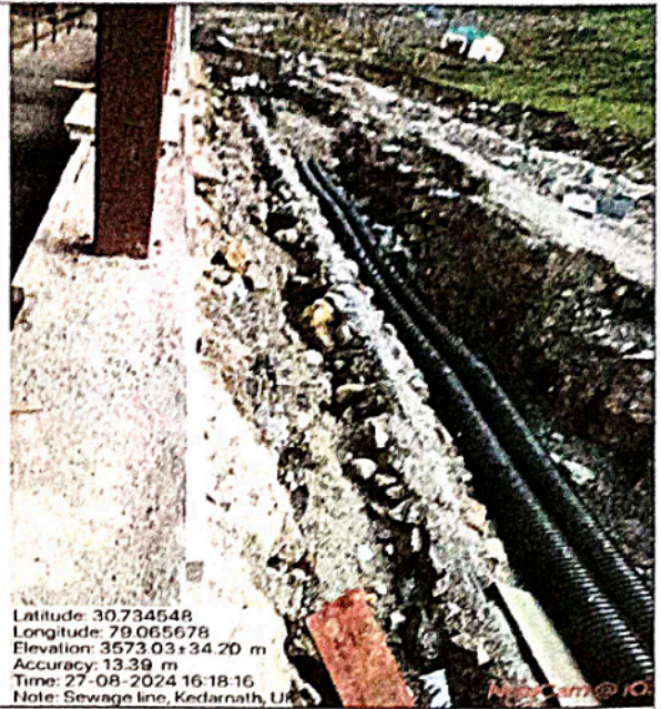
Pic.-6: Construction of sewage lines
