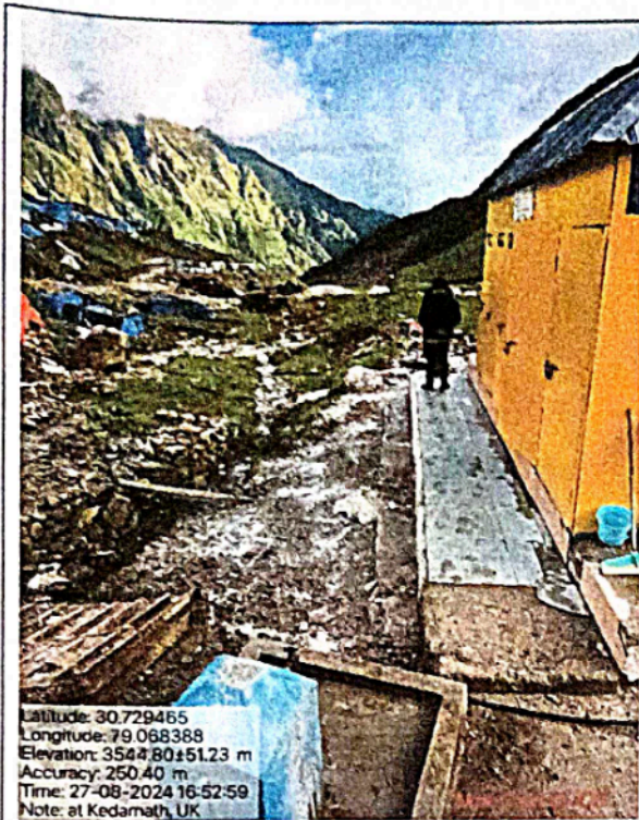
Pic.-9: Seepage of sewage observed near overfilled soak pits.
