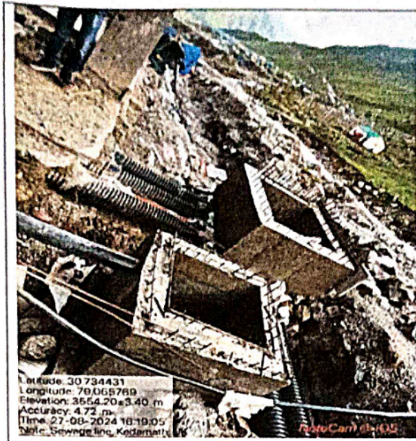
Pic.-5: Construction of sewage lines
